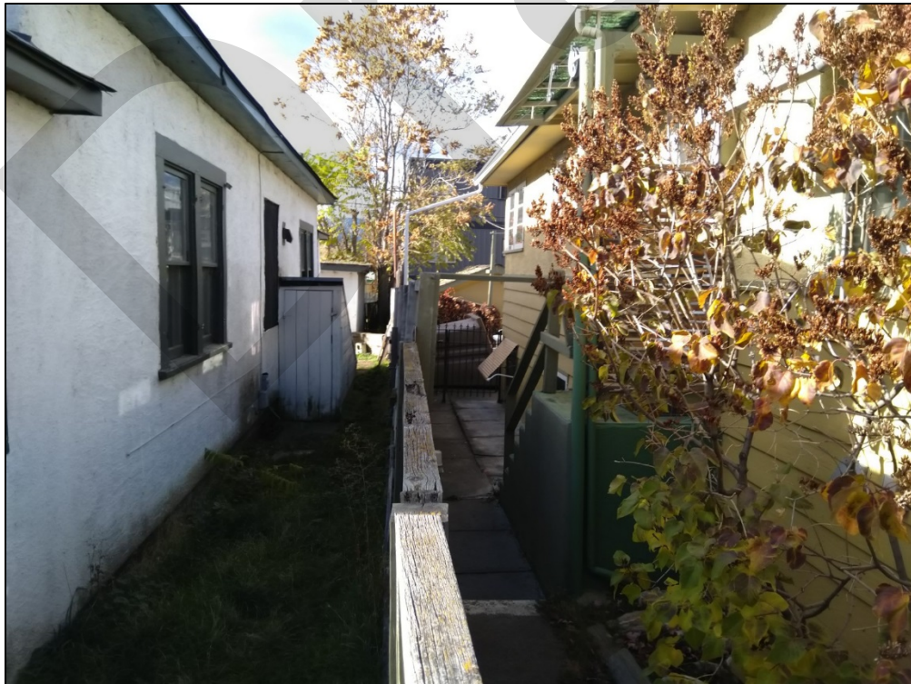
Figure 7: East View showing proximity to north neighbour
