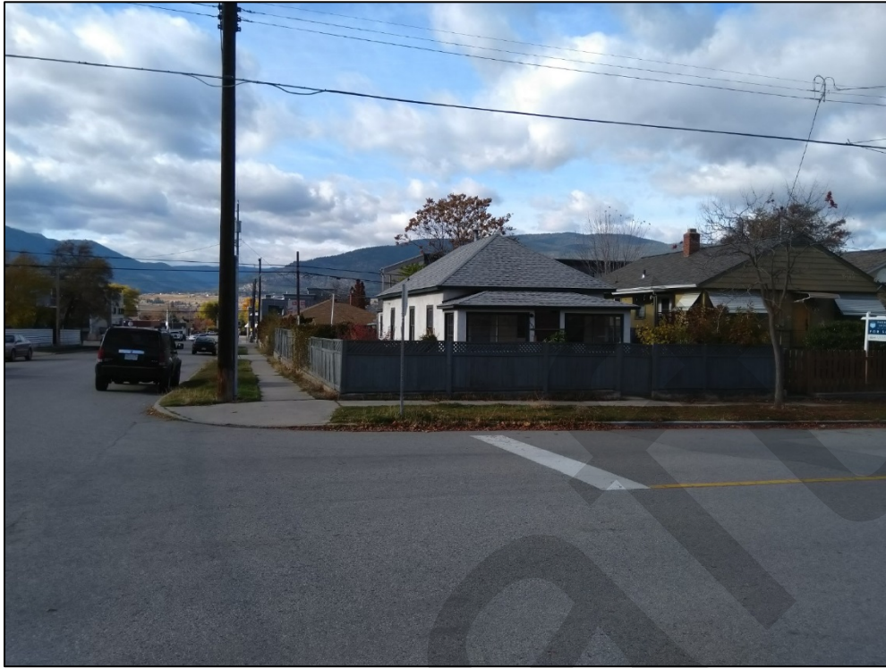
Figure 4: East View (from Van Horne Street)
